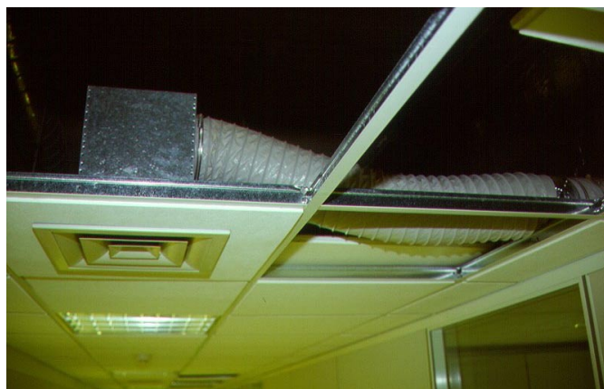
Figure 51: Registers connected to ductwork by plenums.
