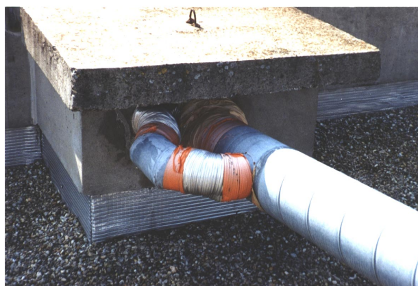
Figure 35: Photograph of poorly installed duct connections.
